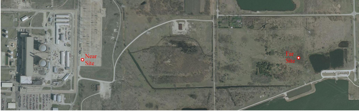
Figure 1: Aerial photograph of the Braidwood Nuclear Power Station showing the locations of the near and far investigative bore holes. The bore holes were located at the proposed shaft sites.
